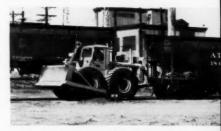
Equipped with railroad coupler, versatile Tournatractor serves as a SwitchTractor, positions rail cars when not working on dozing chores for a U.S. uranium mine. The SwitchTractor can move 5 loaded cars up a 1% grade.
